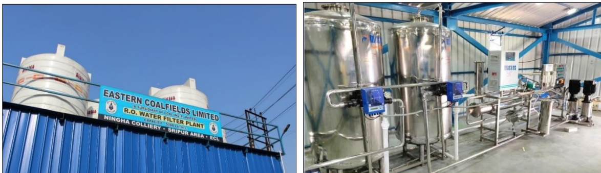
R.O. Filter Plant (120 KLD) installed at Sripur Area, ECL
